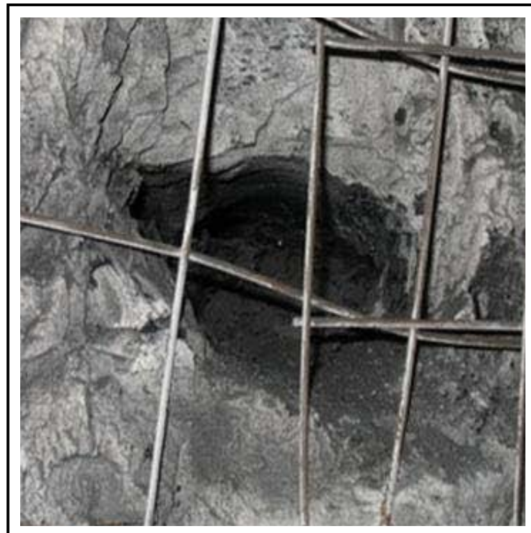
Figure 5.13: Borehole breakout in a UIS borehole at WCC
